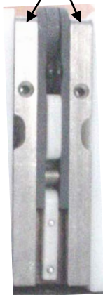
Latch with titanium side bars
